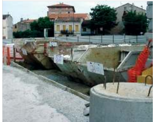
Large containers facilitate sorting of special waste such as timber, window grates, cables and iron.
