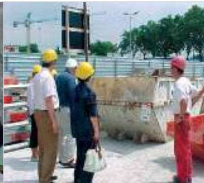
Smaller containers for sorting different types of hazardous and electrical wastes.
