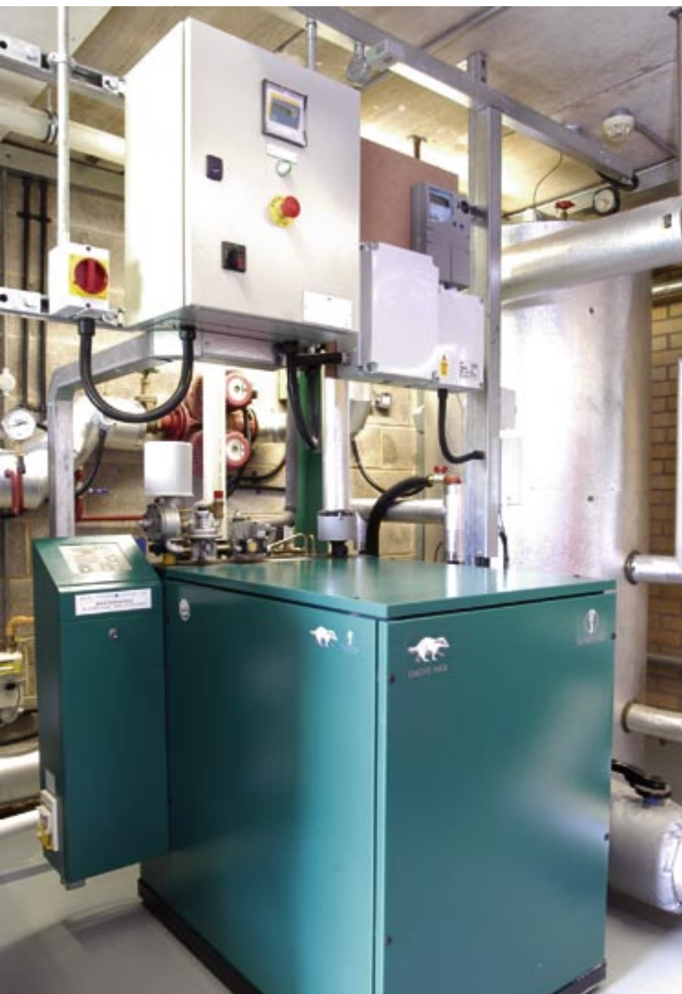
DACHS mini-Combined Heat & Power (CHP) unit at Royal Court, a residential care home in Cheltenham supplied by Bax-Senertec UK, a Baxi Group company.
